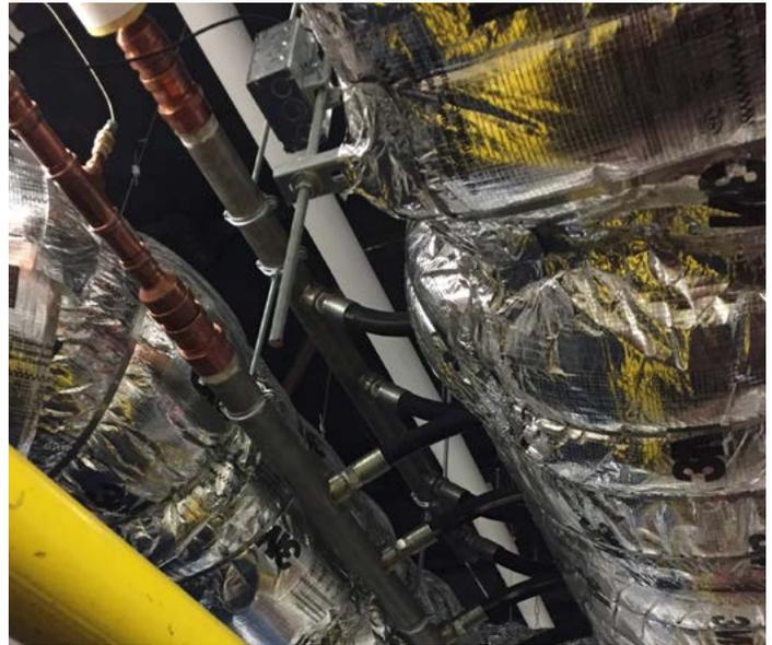
An installed VHX economizer (wrapped in insulation)
